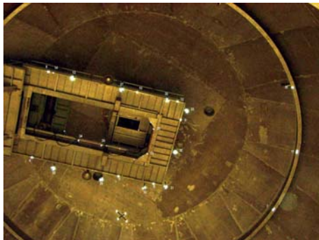
Figure 4a. Resection targets on the crane at the SPF ceiling.
